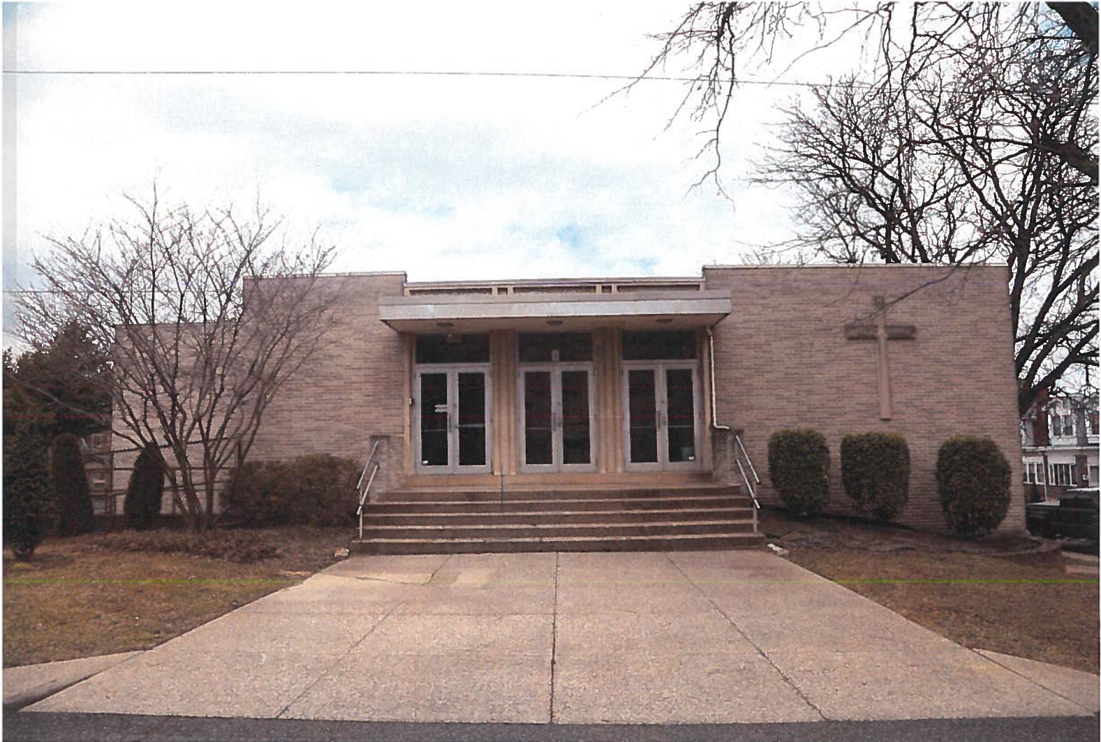
front of building
